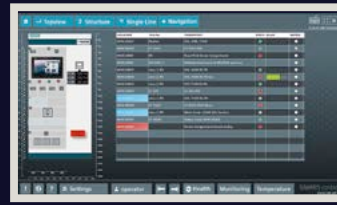
View – individual cubicle
