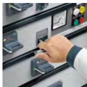
Operating-error-proof and uniform operating concept throughout all sizes of withdrawable units
