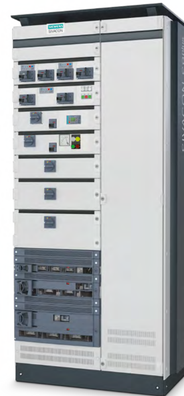
Combination of withdrawable design, fixed-mounted design, and plug-in design
