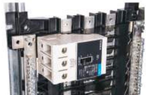
Example of Back-fed NGB Main breaker installed
