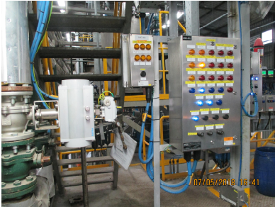
Shutdown valves and annunciator panels installed
