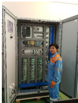
Control panel with FailSafe_Controller, F-Modules
