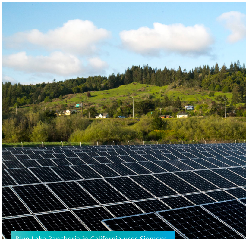
Blue Lake Rancheria in California uses Siemens micro-grid solutions to distributed and control on site power generation.
