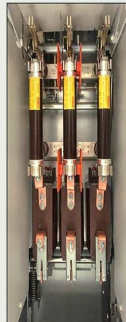
Switch-disconnector/fuse combination
