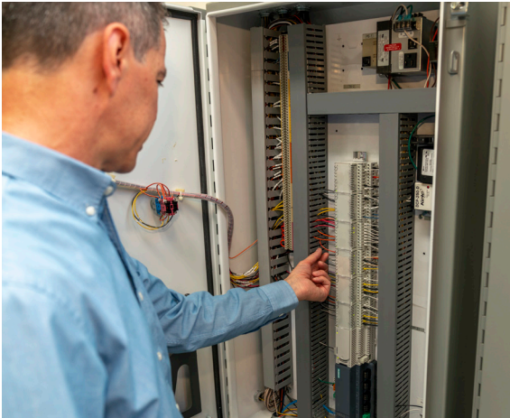
David Carpenter, controls manager, Holbrook Service, (left) inspects control panel with Siemens Designo PXC controller (right)
