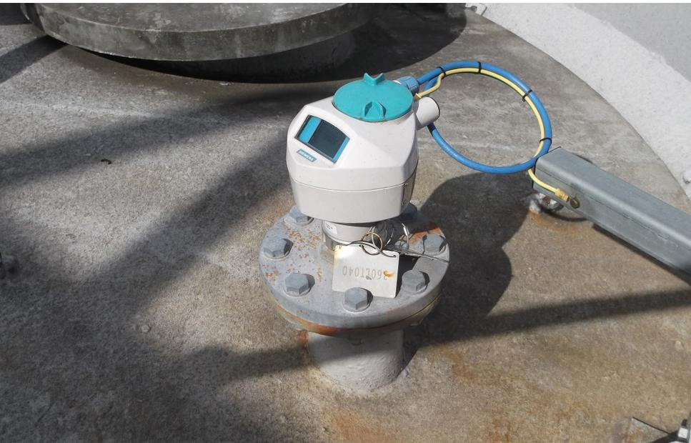
Installing the SITRANS LR250 was easy and PPG now has reliable, high-performance continuous level measurements on their process vessel.
