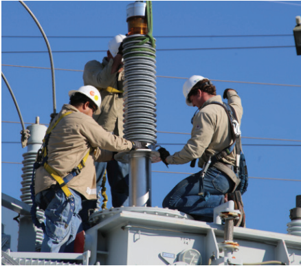
Installation of a 230kV bushing
