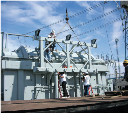
Installation of a cooling system
