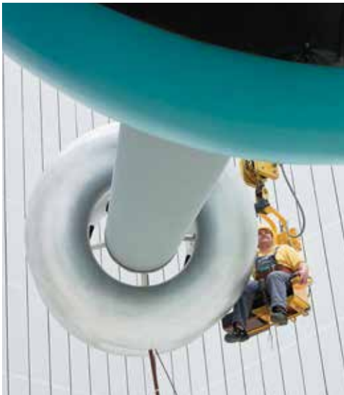
For testing, the transformer is completely set up and connected
