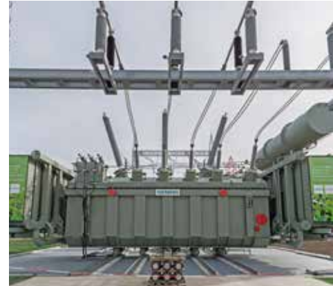
420-kV network transformer with natural ester
