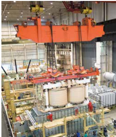
The core-and-coil assembly is lowered into the tank
