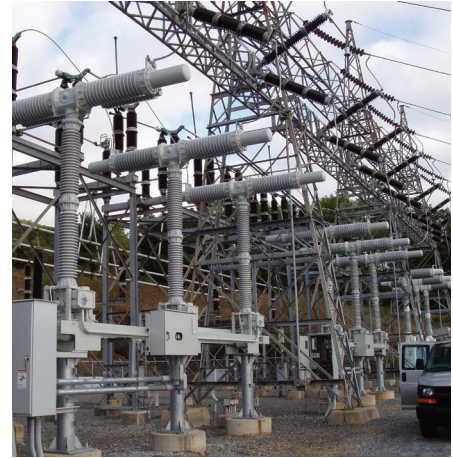
Siemens LPO 245kV live-tank power circuit breaker
