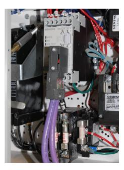
Siemens SIMOCODE has dramatically reduced the wiring required in the motor control centers at Iron Bridge. "You can see how clean this cabinet is compared to the elaborate conduit chases with cables running back and forth in control rooms like this," explained Hester. "Instead a SIMOCODE has been placed in each bucket as a piece of I/O that can easily be added and viewed on the network. It's all part of a totally integrated automation solution that works seamlessly."
