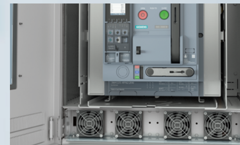
Cooling system with fans underneath the 3WA circuit breaker
