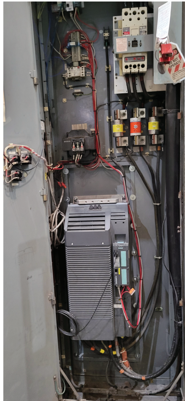
Right: Cooling tunnel fan cabinet with Siemens SINAMICS G120 drive and Power Module installed
