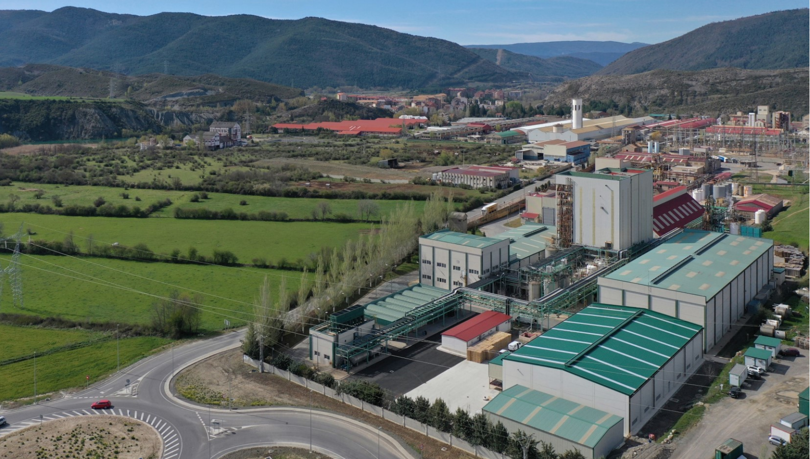
Trouble-free grid operation at the Ercros chemical plant in Sabiñánigo, Spain
