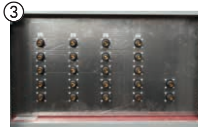
3 2000A example of Crouse-Hinds Cam-Loks for a three phase four wire system with ground connections
