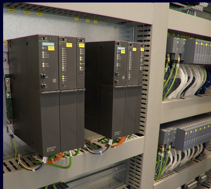
The Siemens process control system operates centrally and independent of local hardware, ensuring updates. Source: Noelle + von Campe
