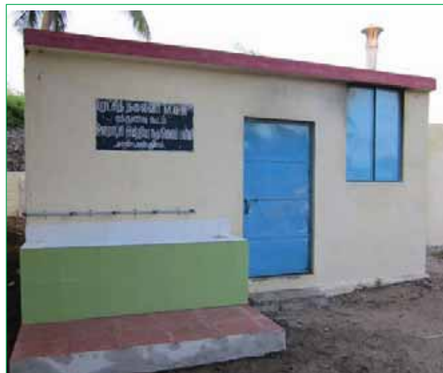
Kitchen shed after renovation.
