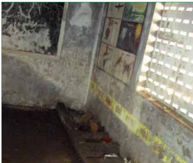
Anganwadi (before) at tsunami-affected village, Tamil Nadu.
