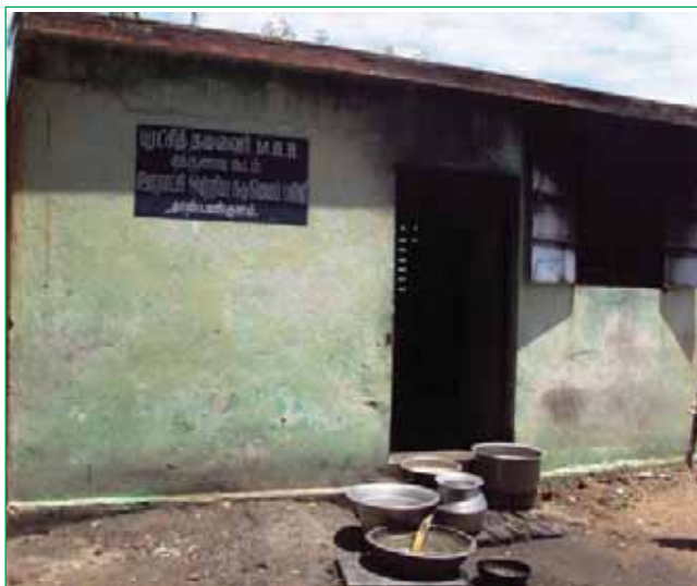
Kitchen shed (before) at tsunami-affected village, Tamil Nadu.
