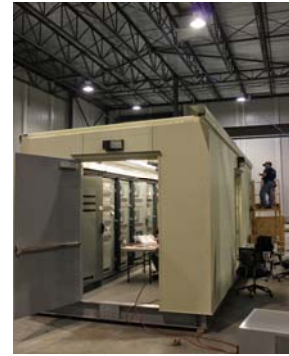
Control Enclosure in construction at the modern Wunderlich-Malec Facility Winslow, ME
