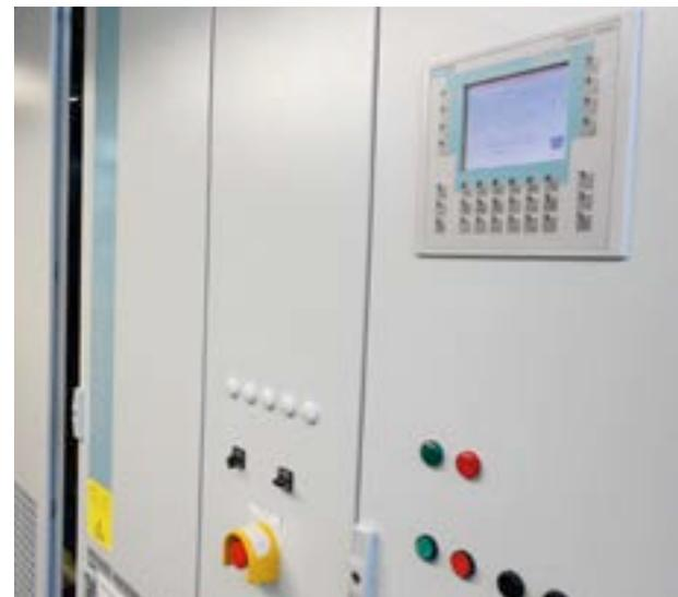
Fig. 2 – SER with SINAMICS S120 converter
