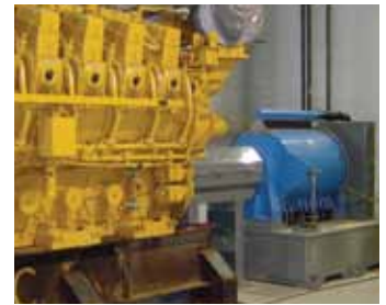
photo credit: Power Test Inc.
