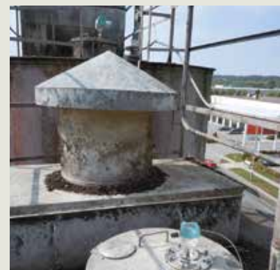
SITRANS LR580 measure the level of malted barley at United Canada Malt Ltd. The compact size of SITRANS LR580 is easy to carry to the top of the silo.
