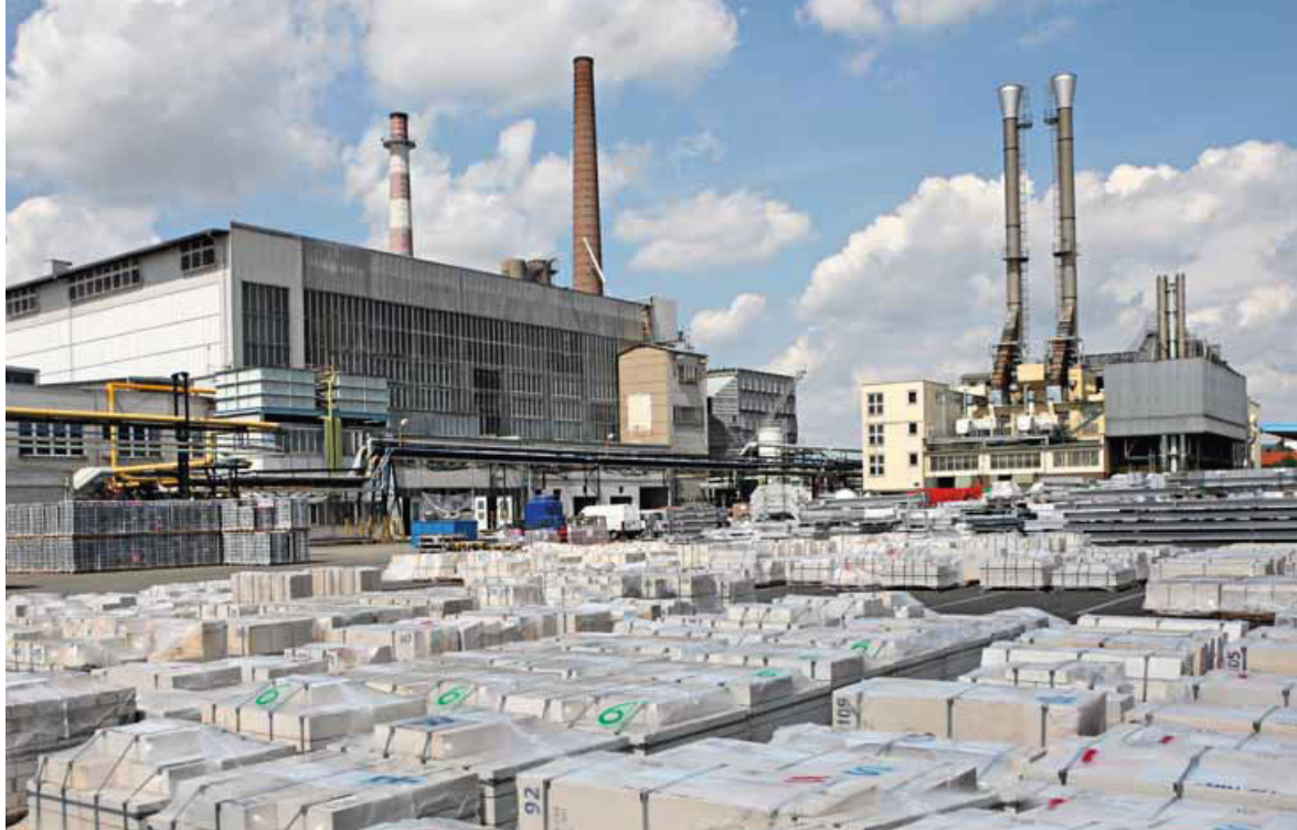
For Vetropack Moravia, HORN Glass Industries planned the entire glass plant with a melting capacity of 350 tons per day
