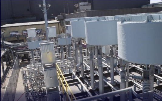
1st Industrial STATCOM, enhancing grid stability
