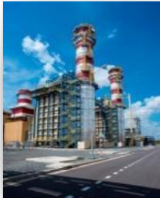
Power island for 750MW Nhon Trach 2 CCPP
