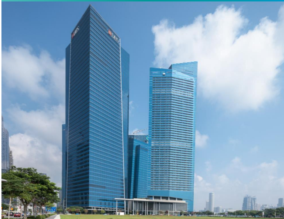
Automation / Fire Safety / Security: Marina Bay Financial Center, Singapore
