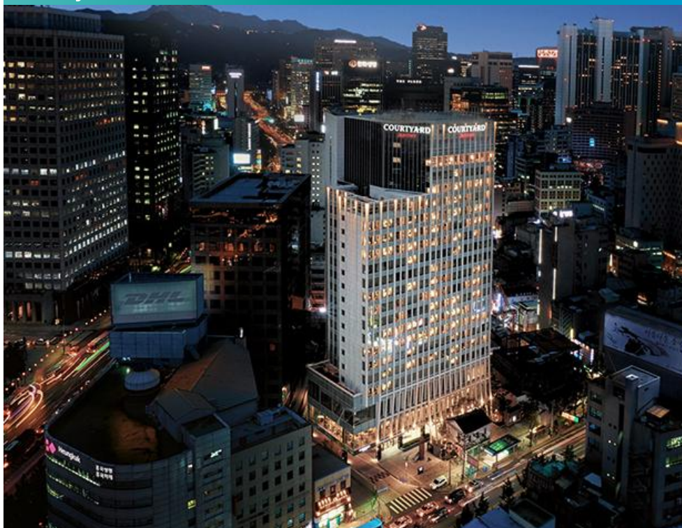
Automation / Fire Safety: Courtyard Marriott Namdaemun
