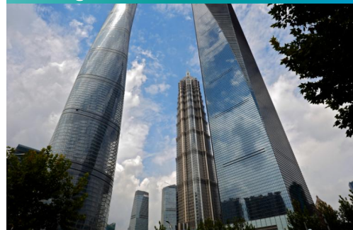
Auto. / Fire Safety: Shanghai Tower, China
