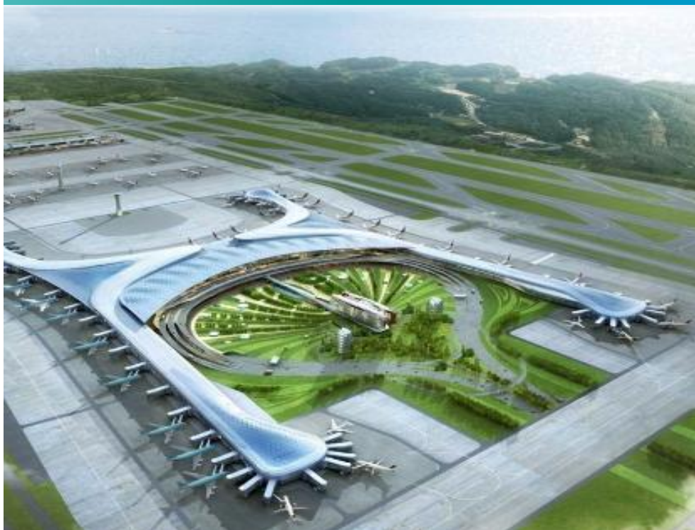
Automation / Fire Safety: Incheon International Airport
