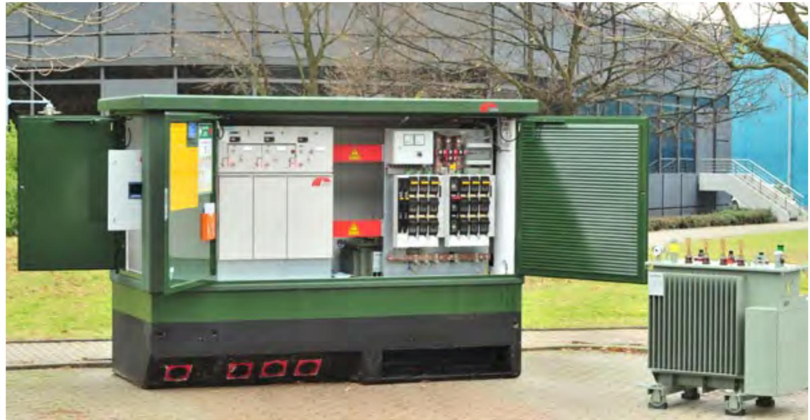
Wachtendonk. The substations are equipped with communication-capable medium-voltage switchgear, adjustable local transformers, and remote-control and distribution grid automation components.
