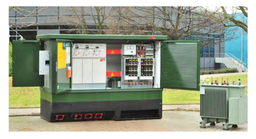
Wachtendonk. The substations are equipped with communication-capable medium-voltage switchgear, adjustable local transformers, and remote-control and distribution grid automation components.
