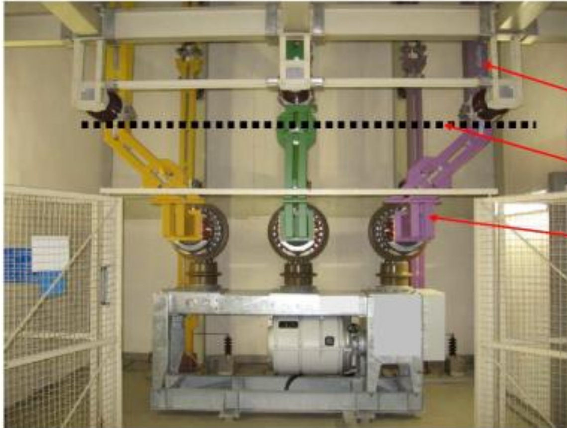
Frontview of the existing SF6-generator breaker ( 24kV – 8500A – 100kA )
