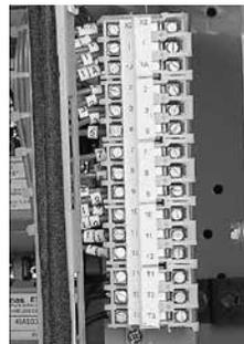
Figura 52. Terminal blocks on swing plate
