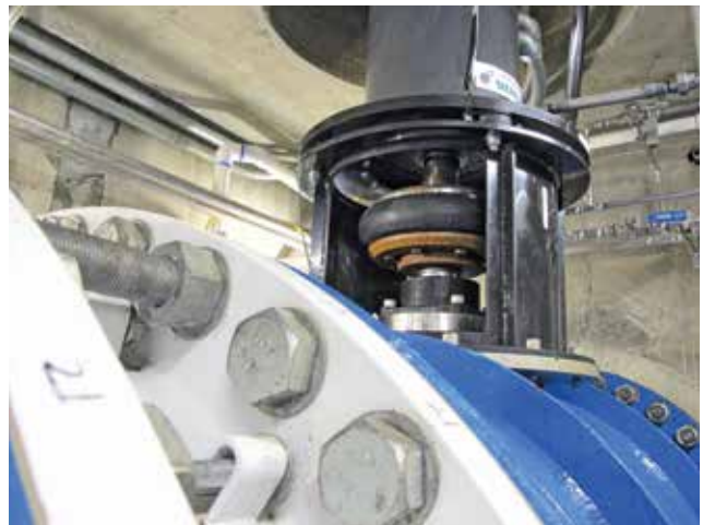
The LucidPipe™ Power System uses a unique lift-based, vertical axis spherical turbine technology to smoothly transfer the kinetic energy of the water flow to rotate the motor shaft without impeding the water flow to any great degree.
