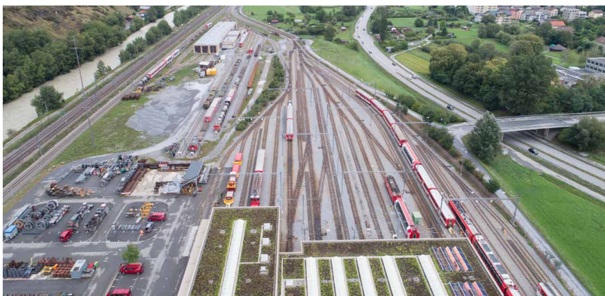
Depot Glisergund, © Matterhorn Gotthard Bahn
