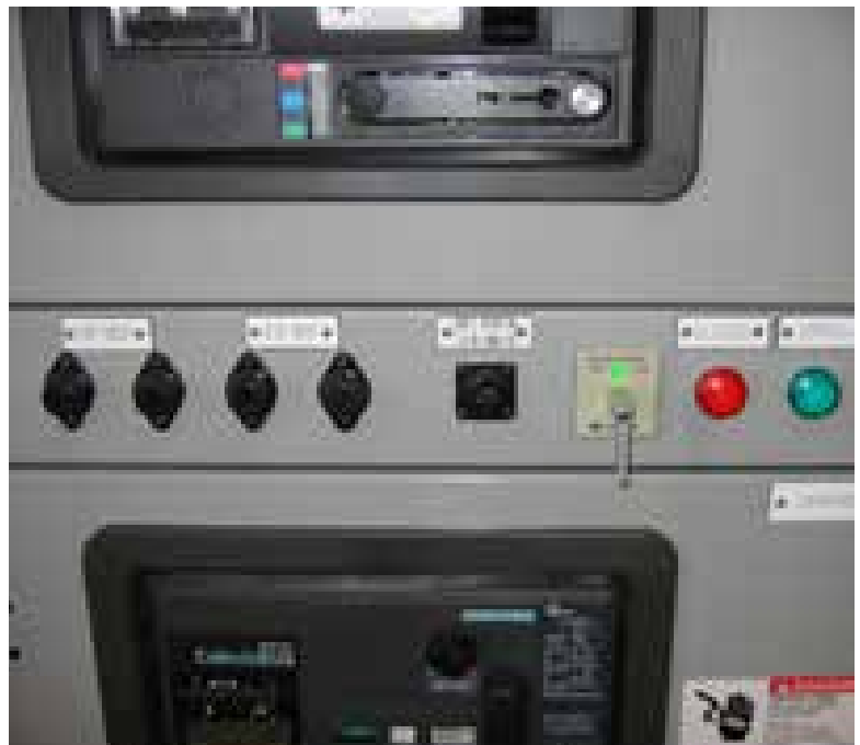
Control port on WL Switchgear
