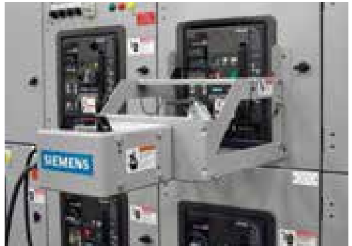
Remote Racking Device
