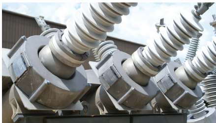
72kV Westinghouse SP breaker
