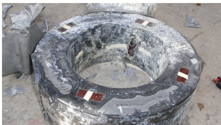
Heavy corrosion on inside of CT housing illustrates the importance of insulation resistance testing
