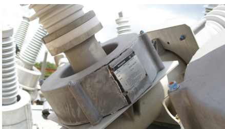
Cracked, weathered CTs on a Westinghouse SP breaker
