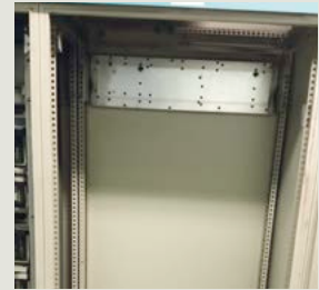
4. Re-align the DC busbar position
