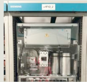
2. Install SINAMICS filter – AIM
