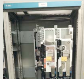
3. Install chassis, connect to DC busbar
