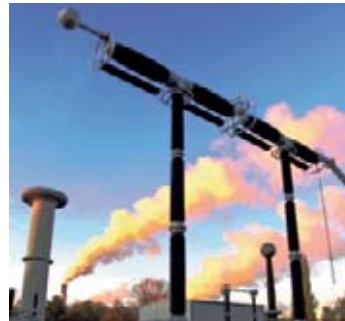
Figure 2: 800 kV live tank circuit breaker
