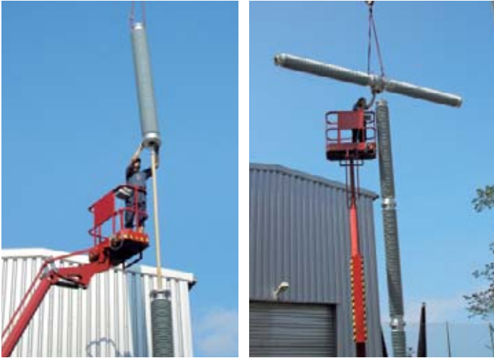
Figure 6, 7: Assembling of the pole column and the double-break interrupter unit
