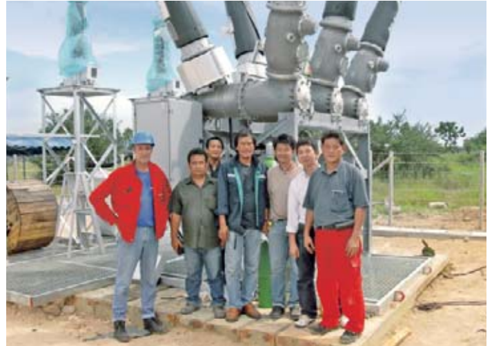
Figure 3: Assembly training for a 3AP1 DTC 145 kV in Thailand
