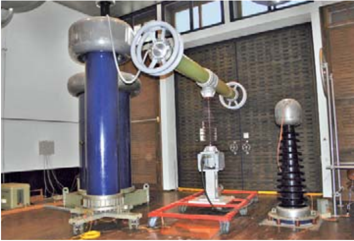
Figure 14: Tests at the Technical University of Munich – measurement of partial discharges under AC voltage
