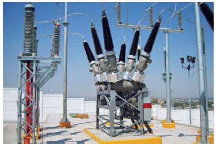
Figure 10: 145 kV dead tank based compact switchgear
