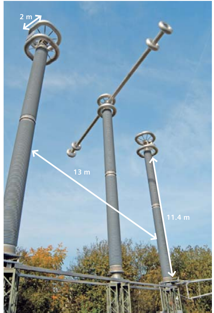
Figure 1: Dimension of 800 kV DC disconnector
