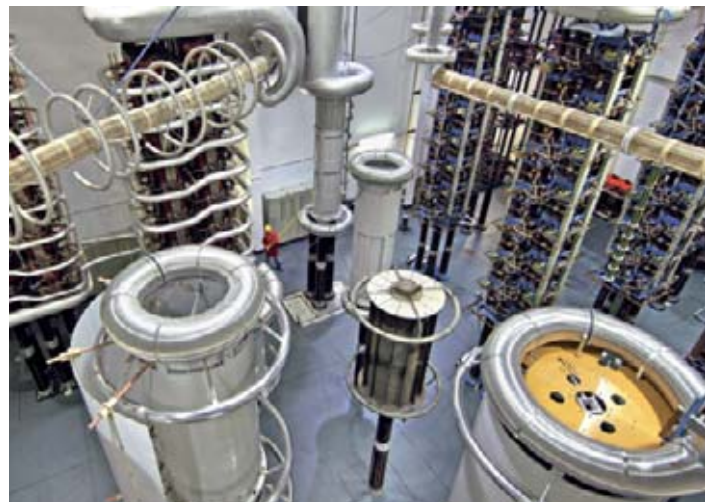
Figure 2: New synthetic circuit after the upgrade in 2005
