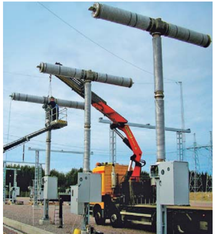
Figure 3: The 3AP2 FI 420 kV DCB on an installation site in Sweden
