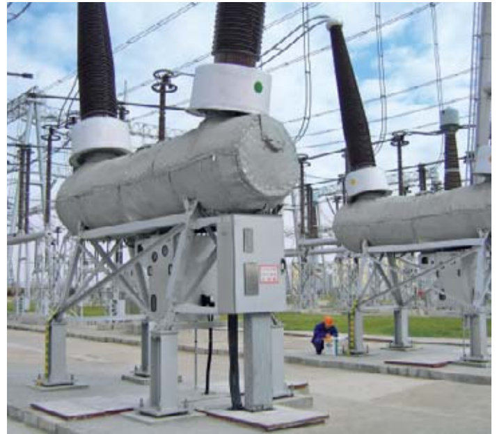
Figure 3: Use of tank heaters and insulation on a dead-tank breaker, type 3AP2DT - 550 kV
