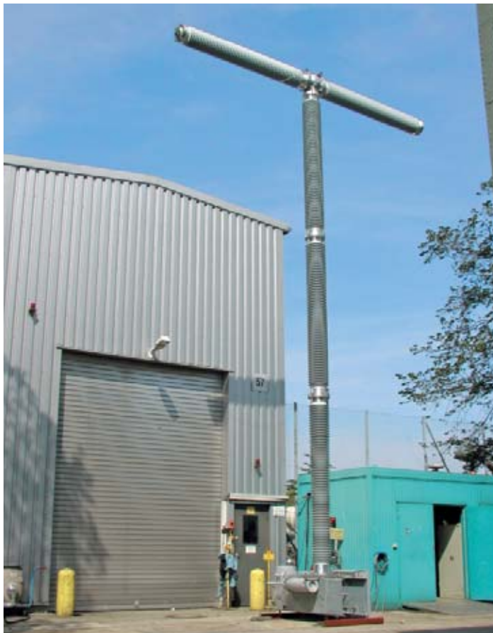
Figure 8: Set-up for mechanical operation tests
