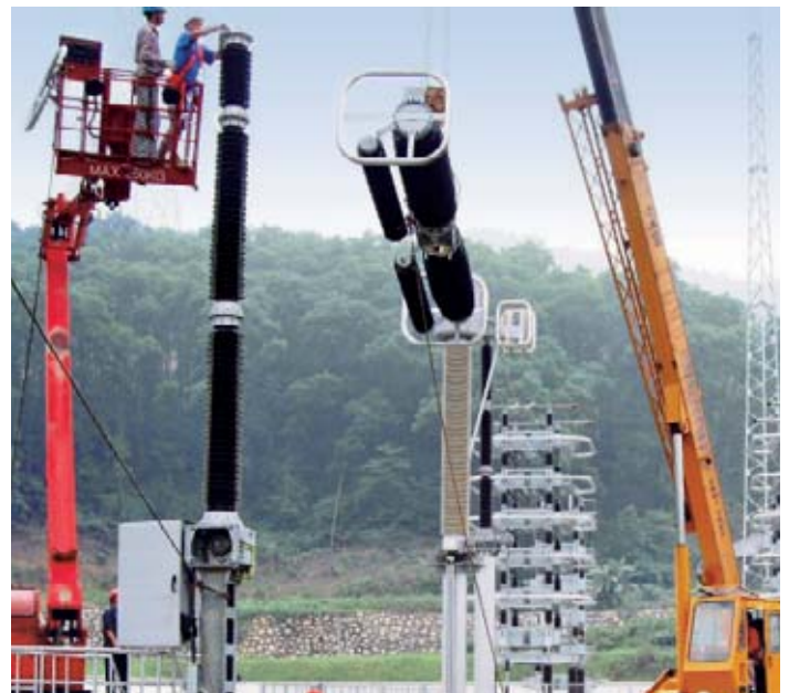
Figure 1: Installation of a 3AP2 FI circuit-breaker for 550 kV in Shenzhen, China
