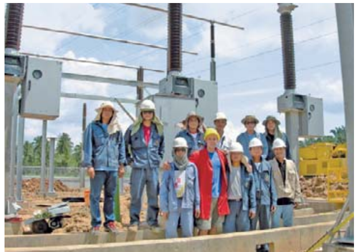
Figure 4: Assembly training for a 3AP1 FI 245 kV in Thailand
