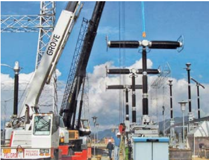
Figure 2: Installation of a 3AT3 EI circuit-breaker for 550 kV in Columbia
