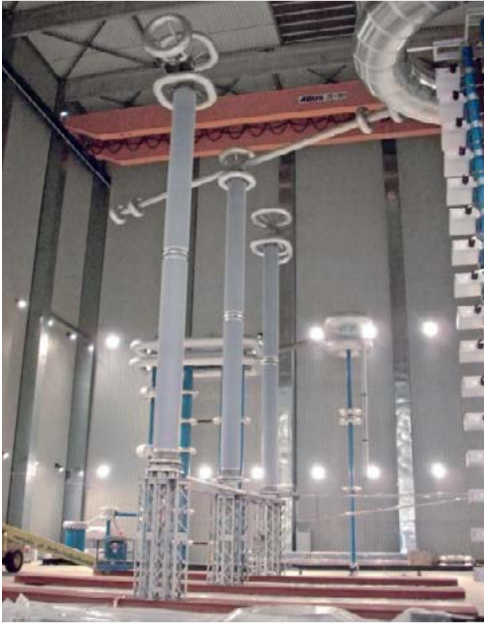
Figure 4: Setup for high voltage tests
