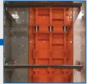
Optional isolated and insulated vertical bus
