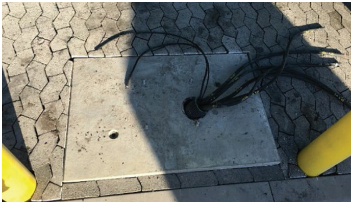
Figure 15: Completed User Unit Foundation Preparation
