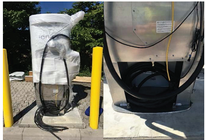
Figure 17: Mounted User Unit, and User Unit Cable Storage (Images indicative only)
