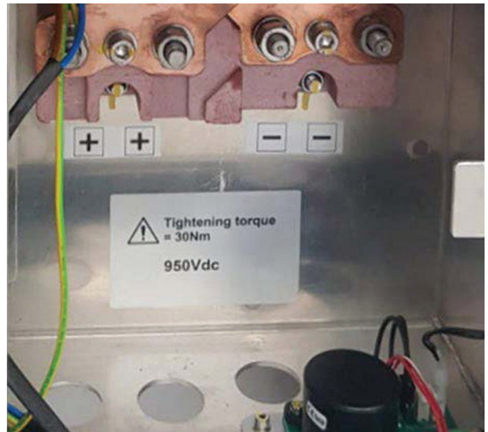
Figure 19: User Unit DC Termination Point
