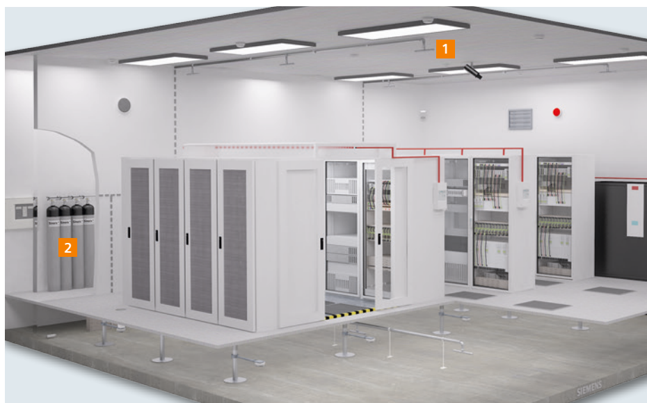
1 Sinorix Silent Nozzle, 2 Sinorix CDT cylinders
