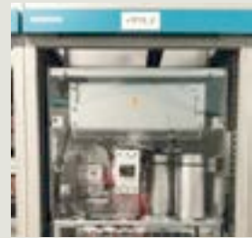
2. Install SINAMICS filter – AIM
