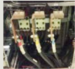
4. Connect motor cables and communication wiring
