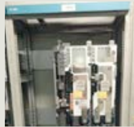
3. Install chassis, connect to DC busbar
