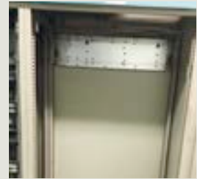
4. Re-align the DC busbar position
