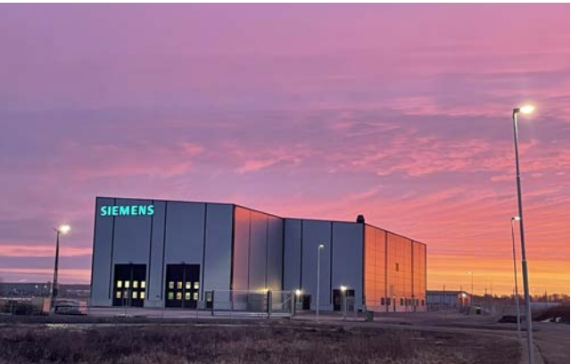
The Rail Service Center in Hallsberg, Sweden, went into operation in October 2022, making it one of the latest additions to Siemens Mobility's depot and service network. The center's experts provide locomotive maintenance, with a focus on overhauls and accident repairs.
