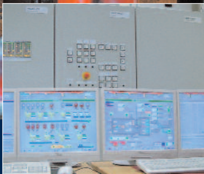
PCS 7 provides the plant operator with all important data
