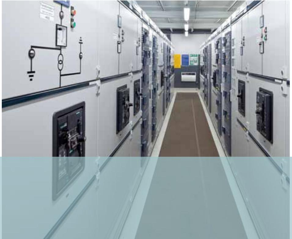
***Sivacon S8 switchgear – in Switchgear Building 6 at ThyssenKrupp Electrical Steel – offers tested personal and plant protection even under arcing fault conditions***
