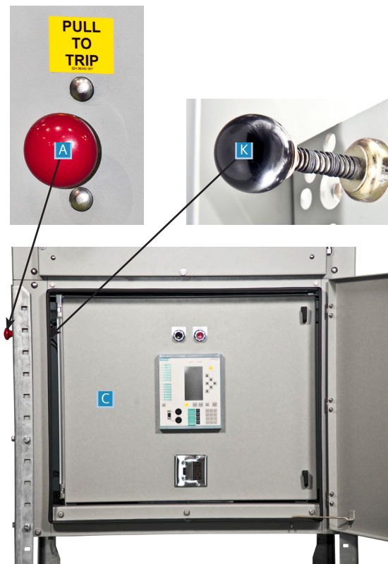
Figure 6: Relay and control and operator compartments for type SDV7-SE circuit breaker with stored-energy operator
