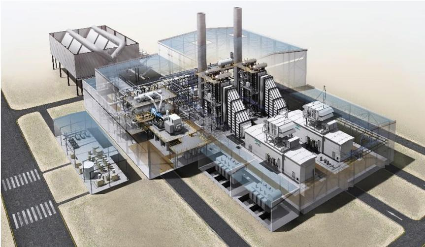
Model showing the new, highly efficient combined cycle power plant that Siemens Energy is going to build in a resembling form at the Marl Chemical Park.
