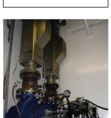
NSB uses Siemens Coriolis mass flowmeters to control and supervise the bunkering process of HFO on the CMA CGM VELA, saving money with every bunkering
