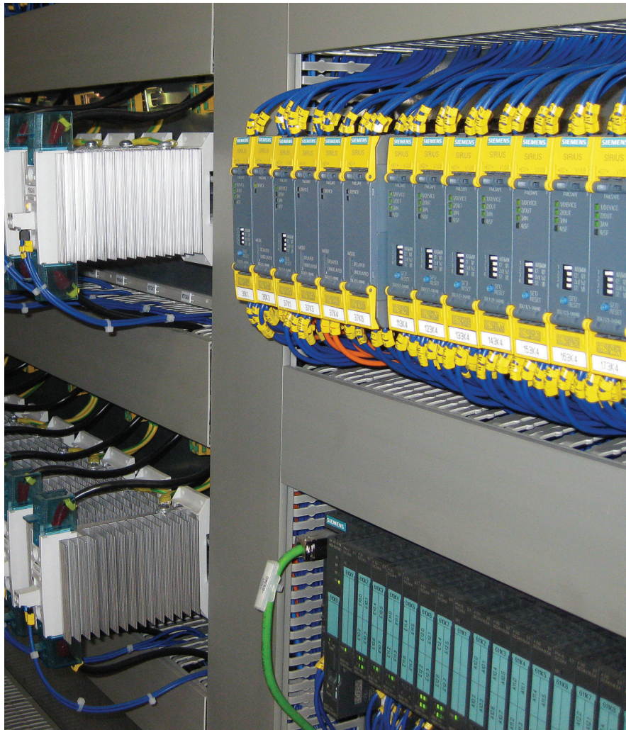
Figure 1 The monitoring and control scheme for Schwartz heat-treatment furnaces features multiple IO-Link masters per furnace, located on the ET 200S distributed I/O from Siemens and connected with the controller via PROFINET.
