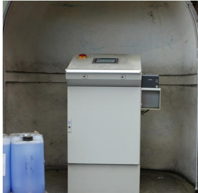
Ergonomic operation: A Simatic Panel as stationary control unit can be found directly above the control cabinet.
