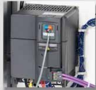
MM4 variable frequency drive with PROFIBUS-DP communication port
