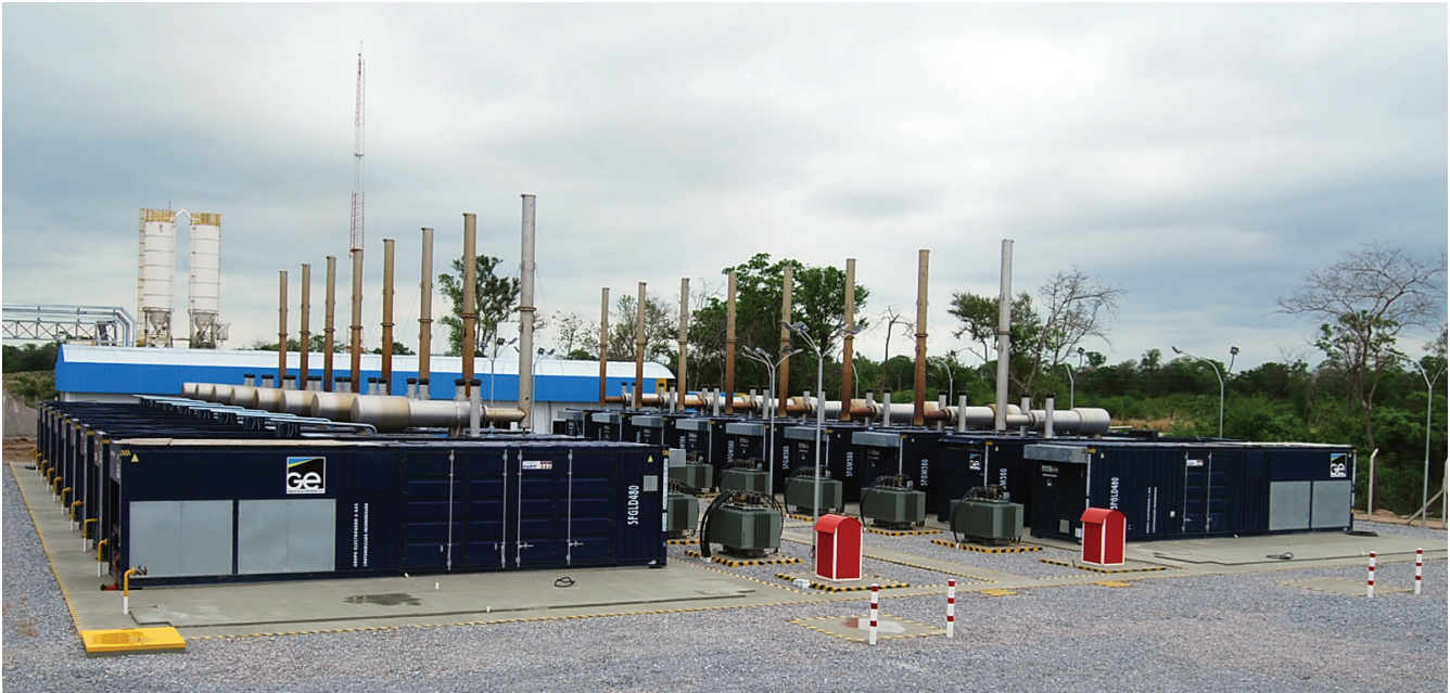
The plant of Itacamba is located in Yacuses, Bolivia, approximately 500 km (311 miles) from the country's capital of Sucre.
