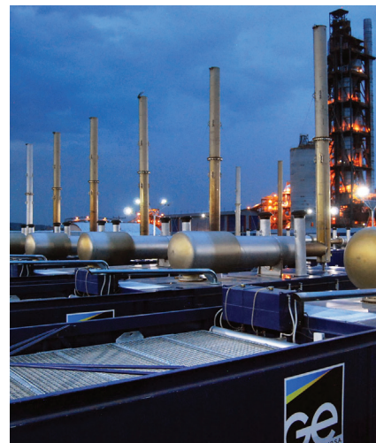
Siemens delivered 16 SGE-56SM (SFGM560) natural gas containerized gen-sets to Brasileria-Boliviana.
